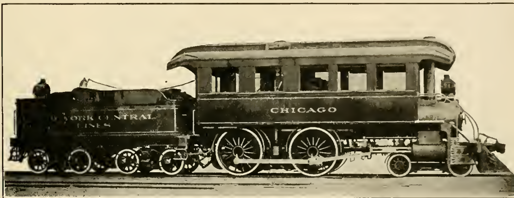
INSPECTION LOCOMOTIVE FOR THE NEW YORK CENTRAL LINES.
